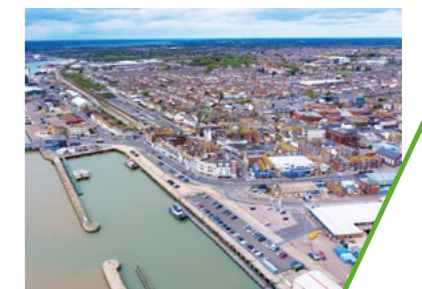
Peterson solidifies its base at ABP Port of Lowestoft
