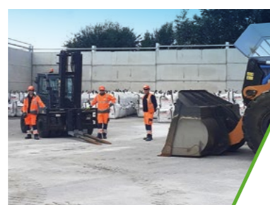
ABP invests £4 million in new equipment, staff, and welfare facilities at its Port of Garston
