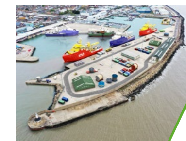
Marine Management Organisation gives consent for ABP's £25 million development of the Lowestoft Eastern Energy Facility (LEEF)
