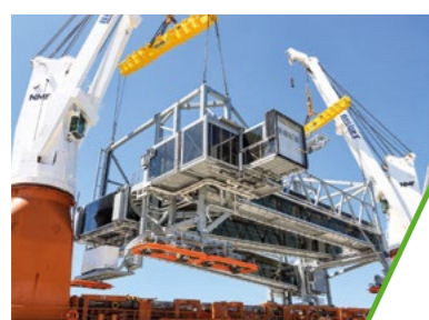
Port of Southampton boosts quayside infrastructure with new airbridge
