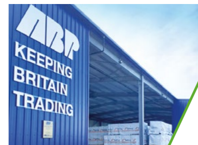
Vancouver Timber Terminal, ABP's £1.4 million Dutch Barn for timber, officially opened at the Port of Kings Lynn
